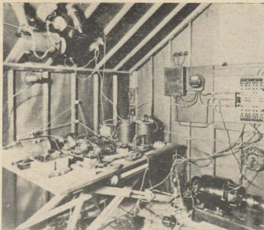
The IBCG M.O.P.A. transmitter. A UV-204A oscillator drove three UV-204As in parallel. The motor generator supplied 2000 volts to the plates for a 990 watt input. Courtesy of the Radio Club of America.
